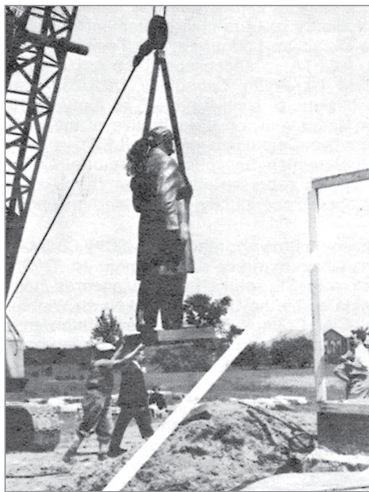
In 1950, a 10'8"-high bronze statue weighing 51 metric tons and a 10'3"-high granite pedestal arrived in 121 pieces. Here, the figure is being hoisted into place by crane. Spring, 1951
